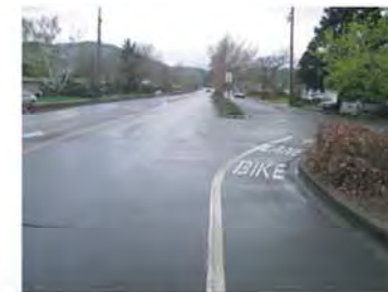
Looking NE down Center Road
