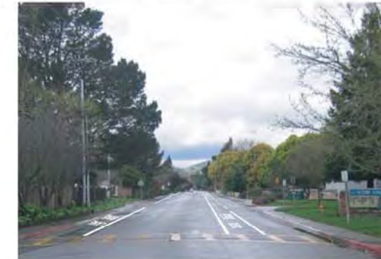
AFTER: Option 3 - Bike Lanes, Parking Both Sides, Restricted Parking During School Hours
