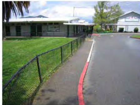
Pick-up drop-off area in front of school. This plan recommends that the fence be moved back 5-10 feet and a taller curb be constructed.
