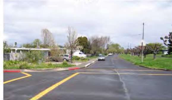
Intersection of Lynwood and Sunset showing current conditions.
