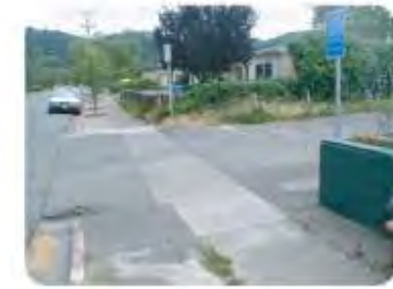
Mohawk Ave. at School Entrance, looking south
