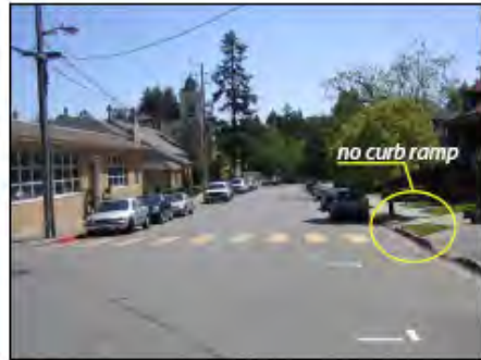
Existing crosswalk on King Street lacks signage
