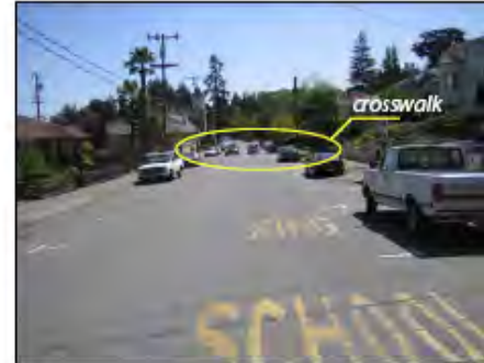
Existing pavement markings on King Street are too far from crosswalk
